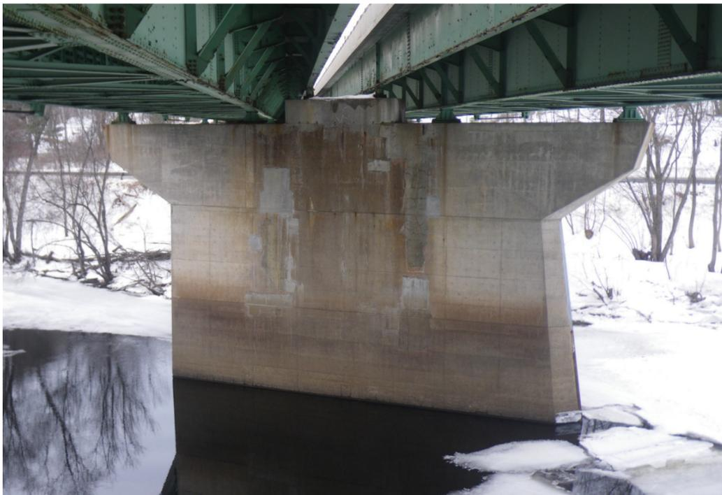
**Figure 2 View of Pier Concrete Deficiencies.**
