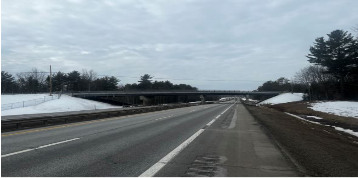
Looking south at the new Route 197 bridge.
