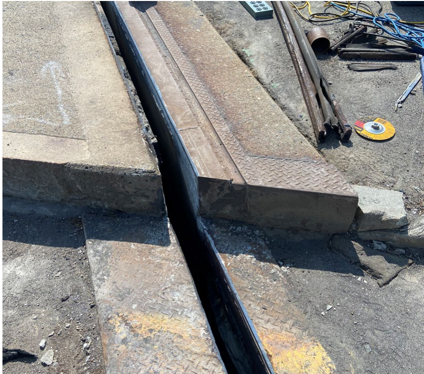
Looking south at the western bridge joint modifications at Route 236
