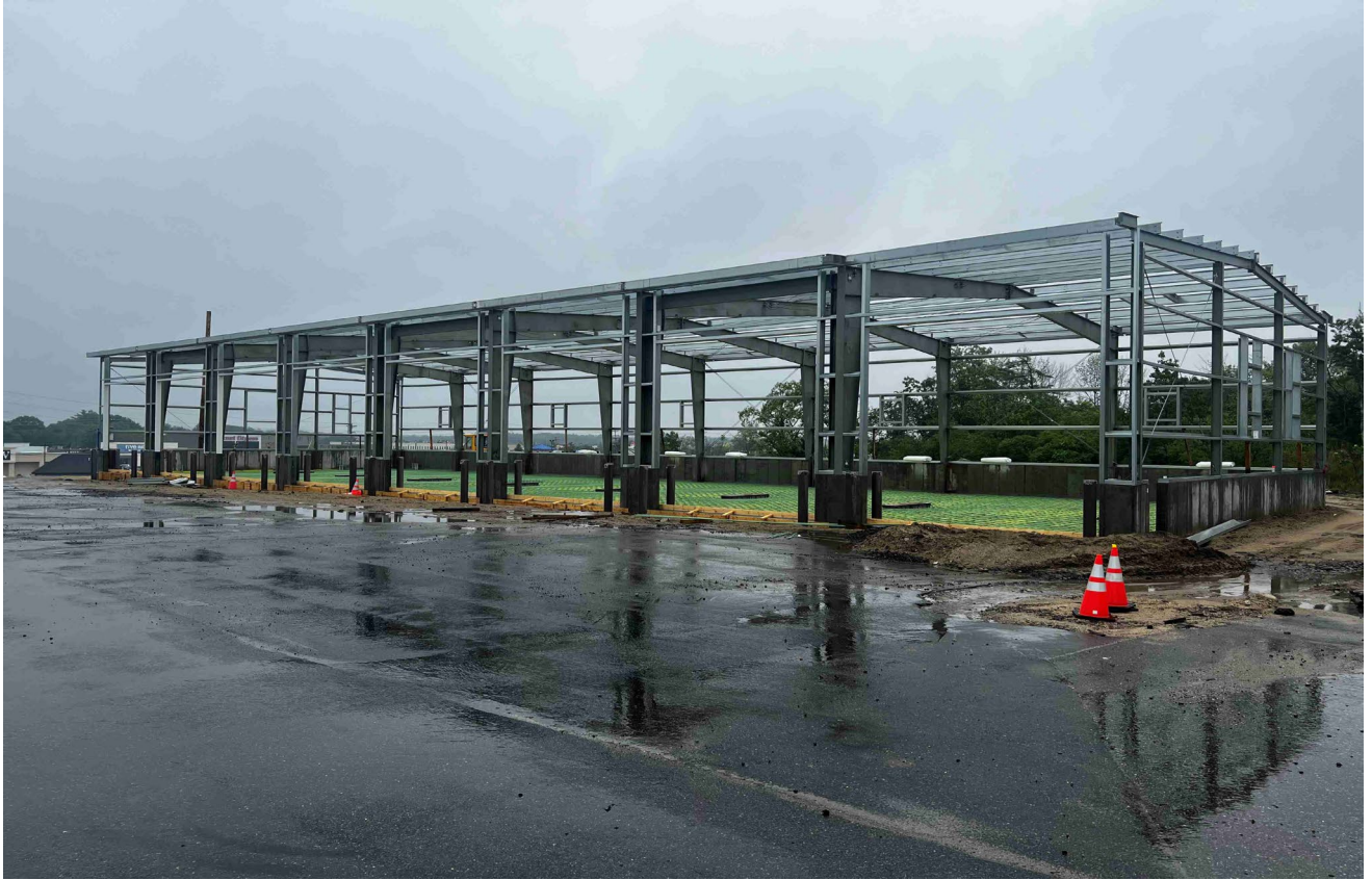
The building is prepped for the concrete slab.
