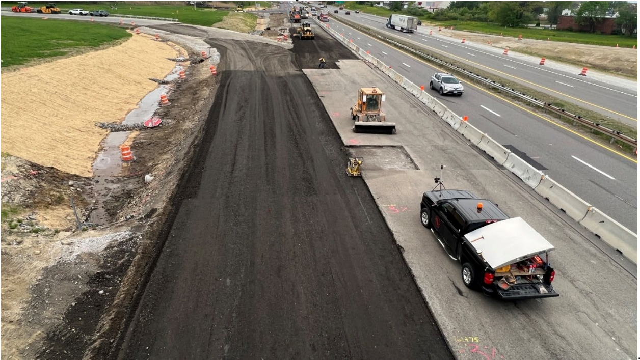
Fine grading during exit 48 northbound on ramp closure.
