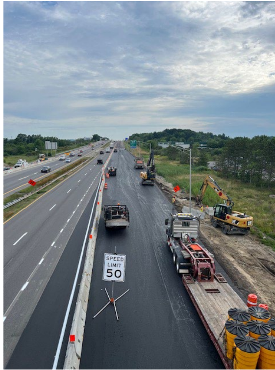
Slope construction along northbound mainline north of Exit 47.
