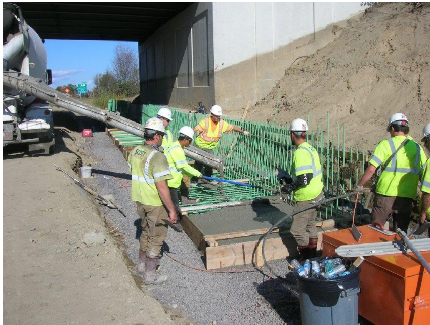
Running Hill road bridge protection
