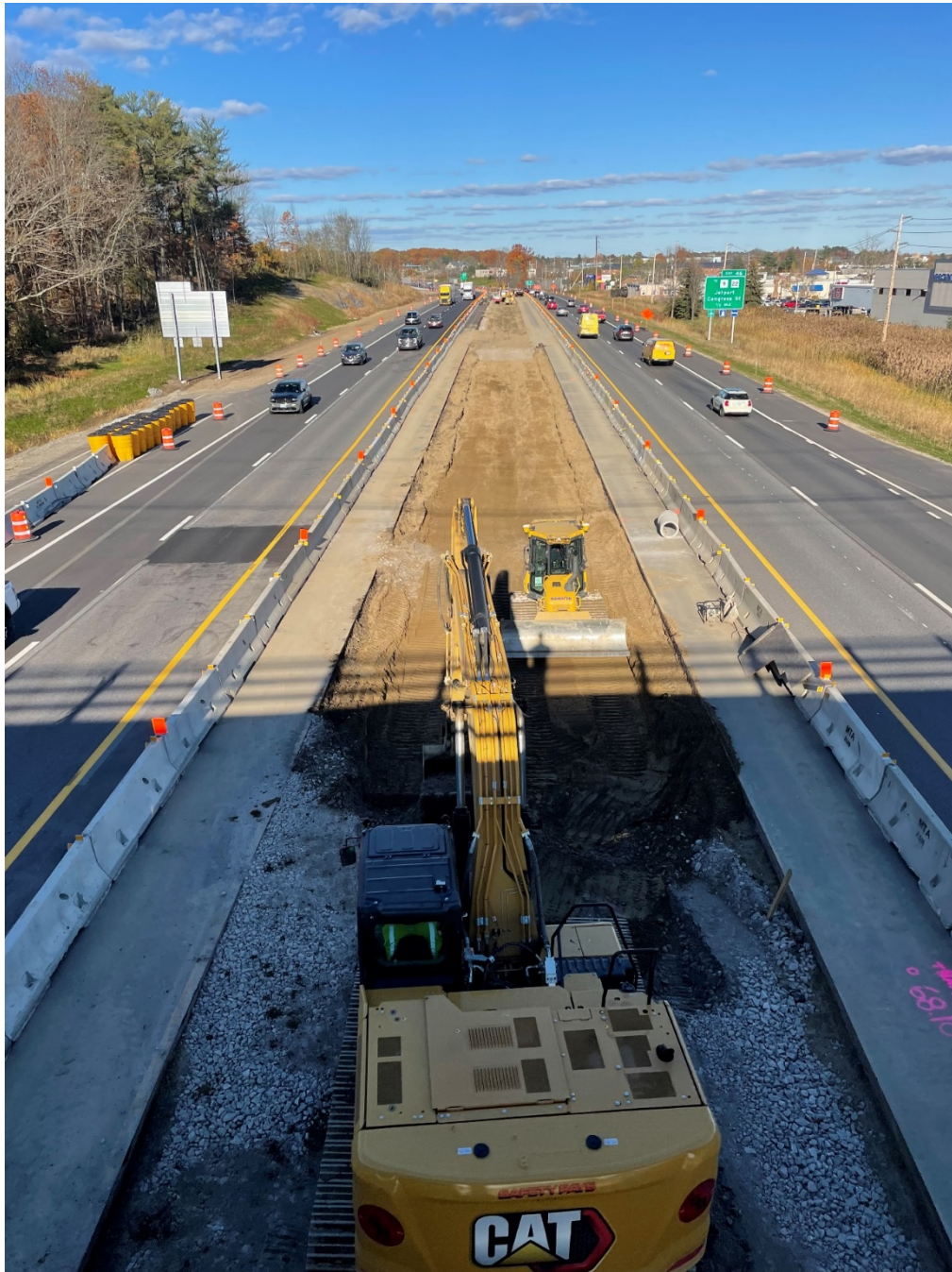
Looking north from Running Hill Road Bridge
