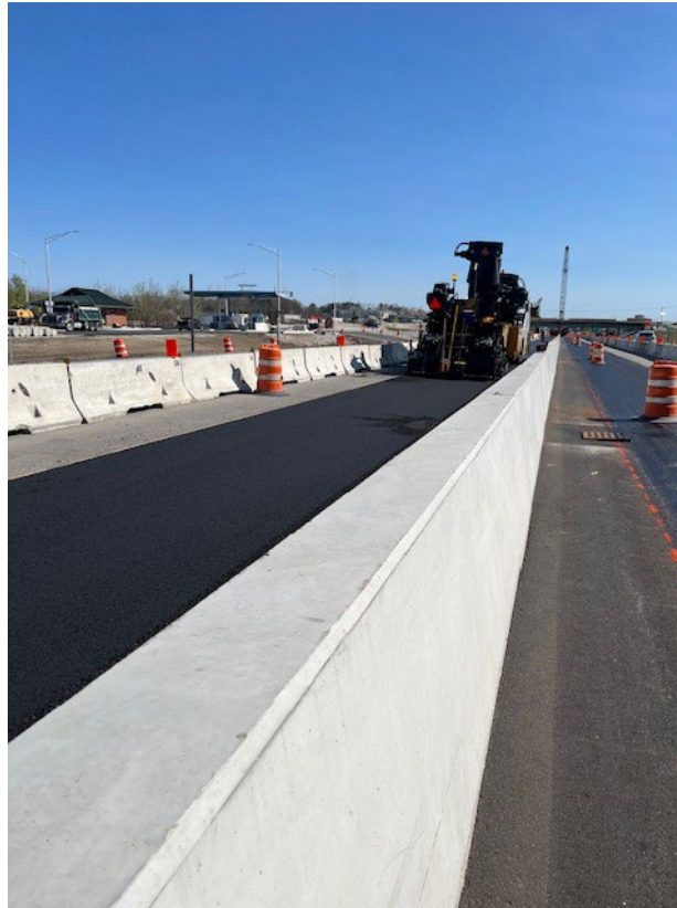
Paving adjacent to the median barrier
