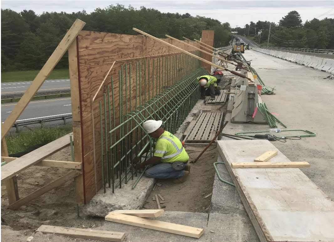
Tying Rebar for the Shaker Road Bridge
