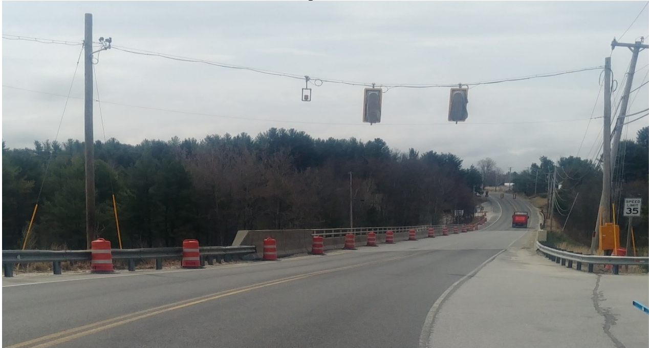
Route 26 Bridge, Looking East
