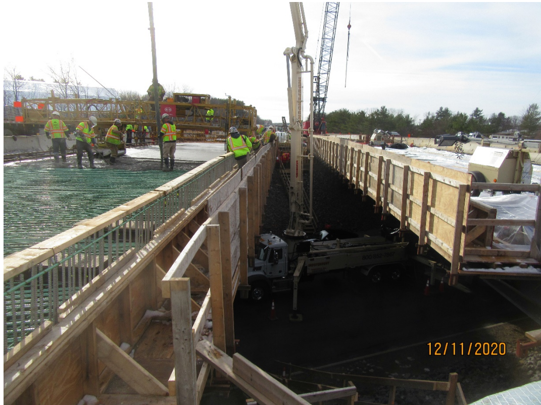
Placing concrete NB deck Warren Avenue
