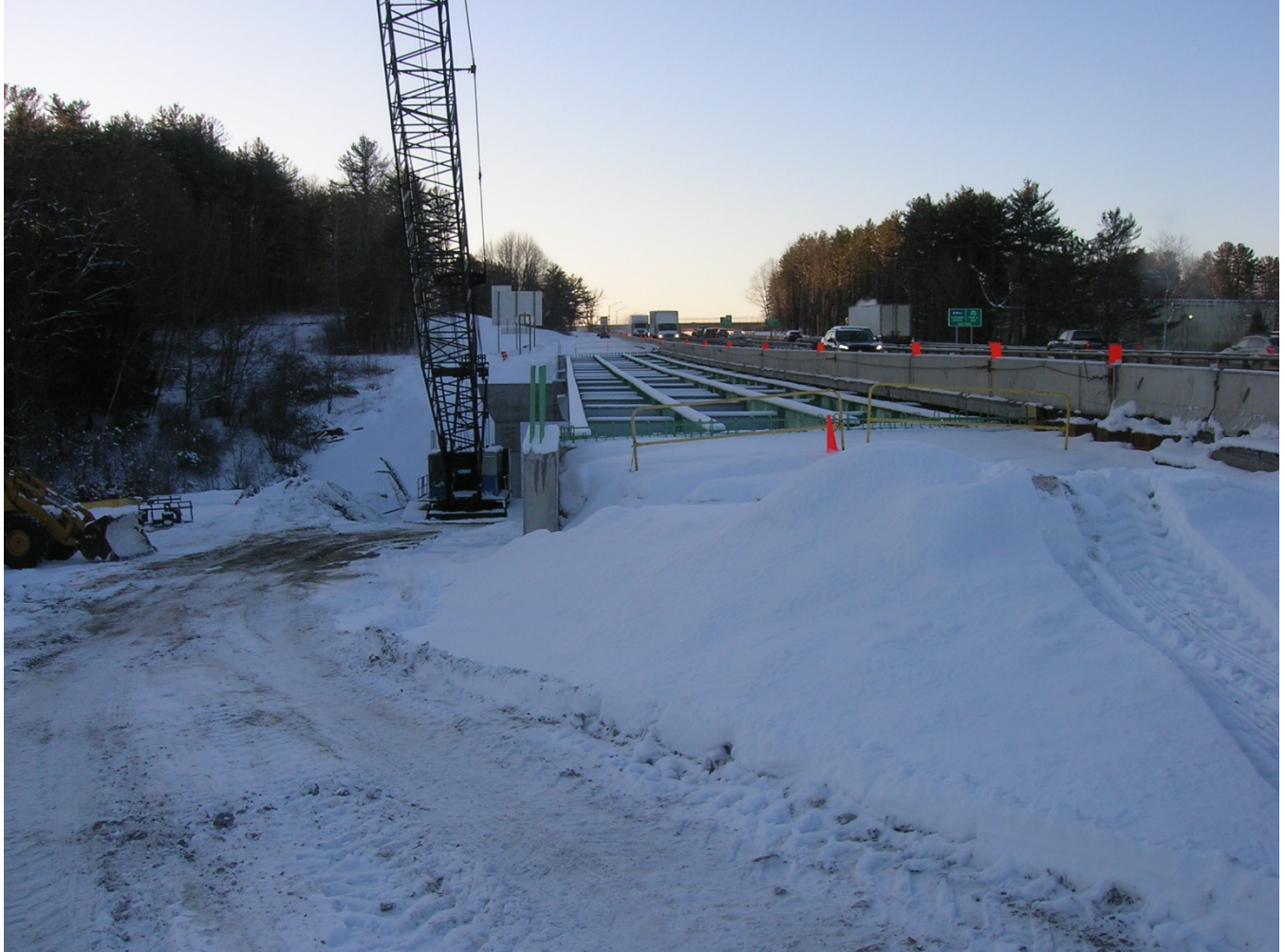
Looking south at Stroudwater Northbound Bridge
