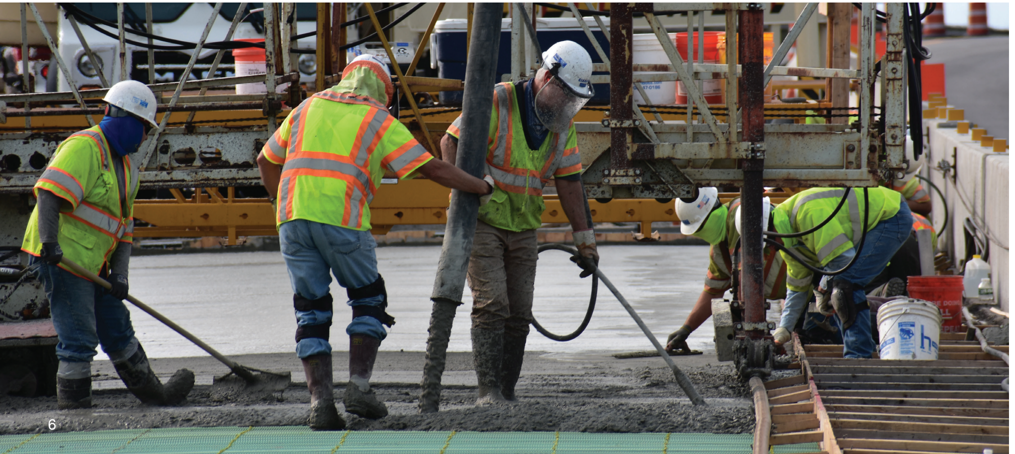
Concrete deck placement at Stroudwater River Bridge in Portland
