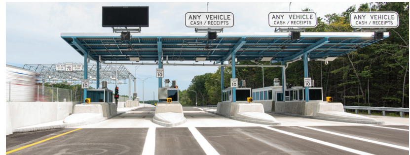
The northbound cash lanes just prior to opening in September
