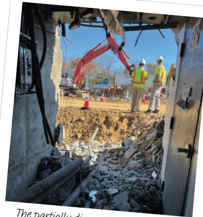
The partially dismantled tunnel at the York Toll Demo Site
