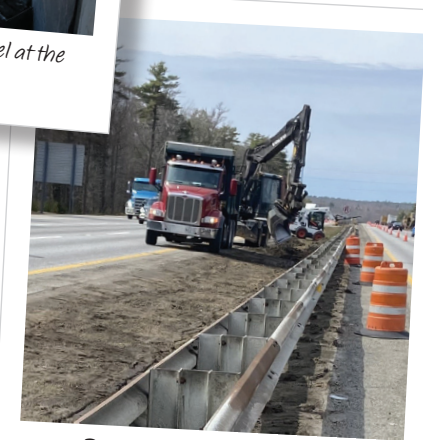
Pavement rehab in Biddeford
