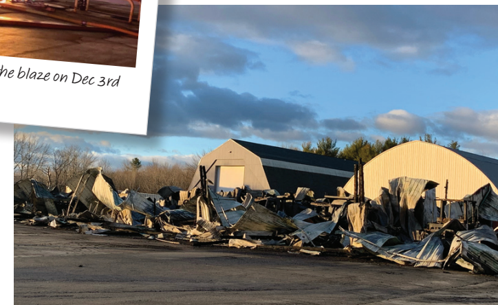
The damage from the fire at Litchfield Maintenance
