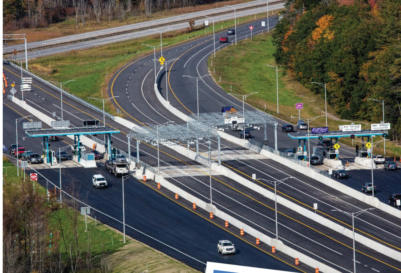
The ORT Plaza almost complete in October
