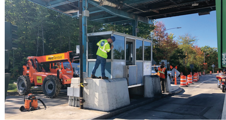
CPM Constructors work to replace the damaged booth
