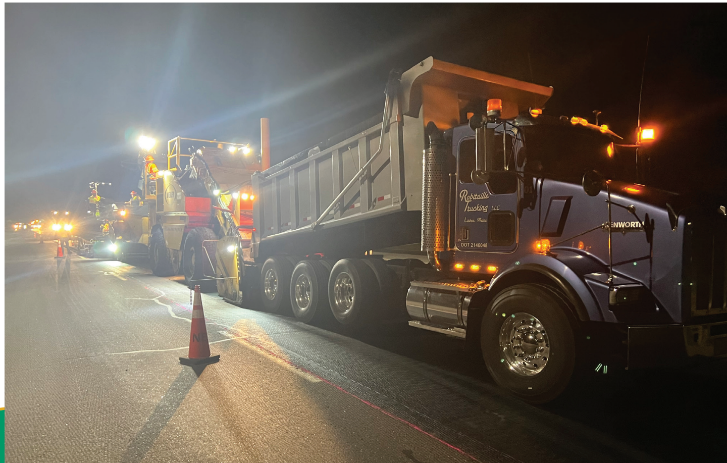
Nighttime pavement rehabilitation in Gardiner
