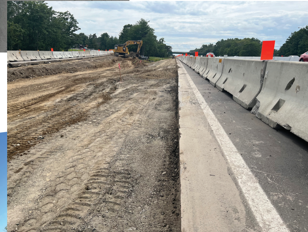
Restoring roadway after toll plaza demolition at Mile 7 in York
