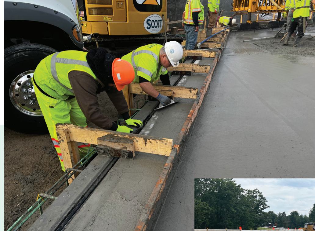
Concrete deck placement at Route 197 Bridge in Litchfield
