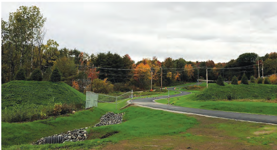
Blackstrap Road EVR Completed
