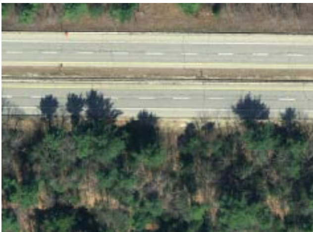
Tree shading on Turnpike before clear zone improvements
