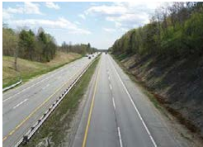
Mile 53 Maine Turnpike after clear zone improvements
