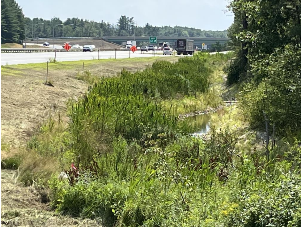
Photo 2 – Unnamed tributary to Thatcher Brook at the Exit 32 southbound off ramp in Biddeford. MTA relocated the stream further from the road in 2021, and has been implementing measures to keep the riparian buffer in an unmowed condition. MTA plans to augment the unmowed riparian buffer with a shrub planting in 2024.
