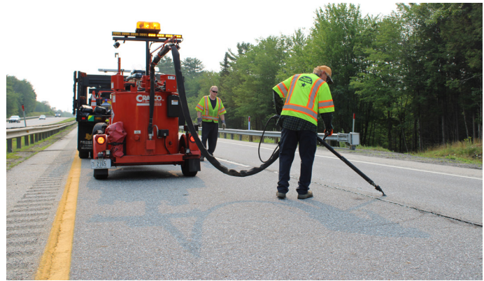
PAVEMENT REHABILITATION BY MTA MAINTENANCE CREW
