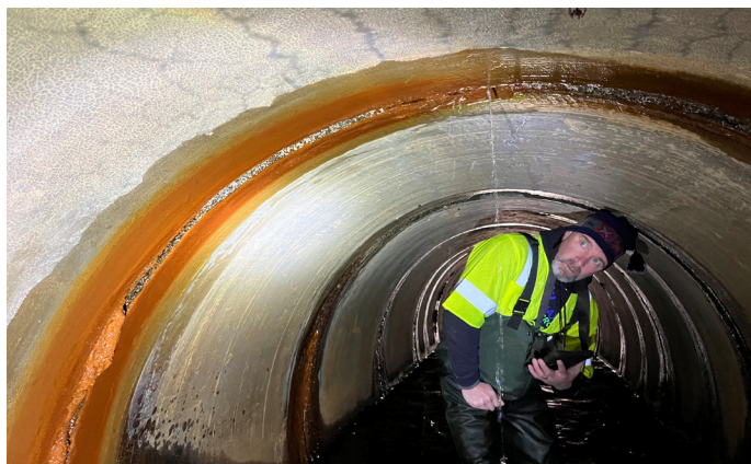
PIPE CULVERT INSPECTION
