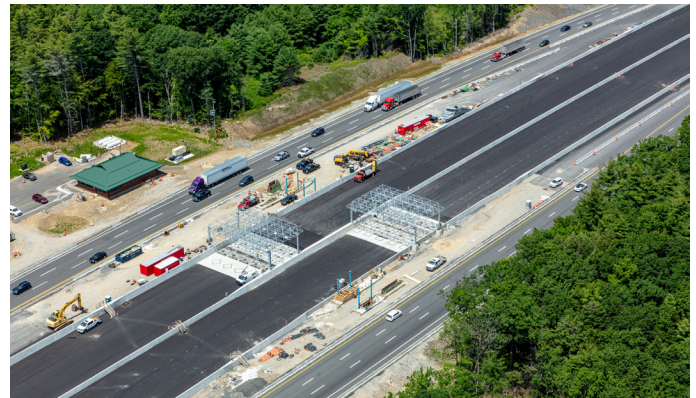
YORK TOLL PLAZA CONSTRUCTION
