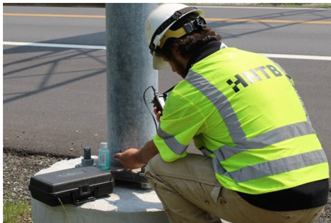
ANCILLARY STRUCTURE INSPECTION
