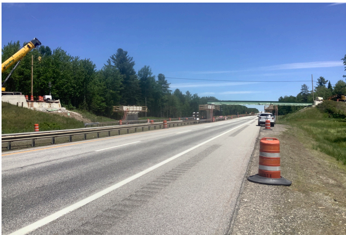
ROUTE 197 UNDERPASS SUPERSTRUCTURE REPLACEMENT
