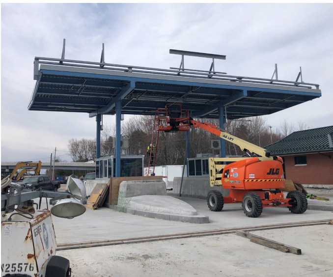
TOLL CANOPY CONSTRUCTION AT EXIT 45 INTERCHANGE
