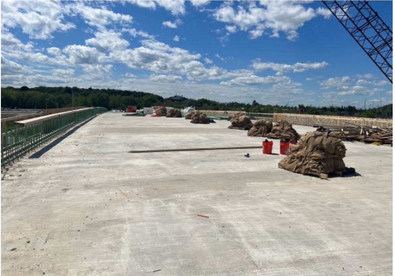
Looking west at the recently replaced exit 45 bridge deck.
