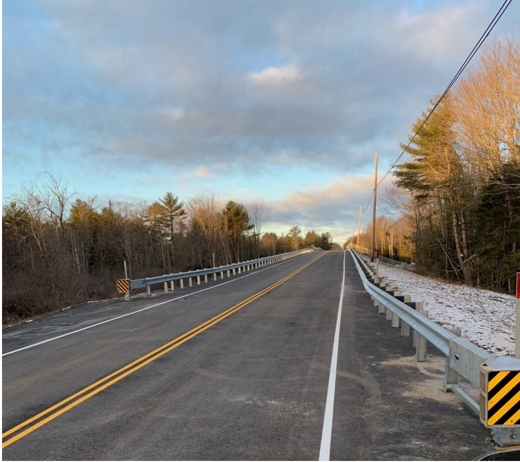
Bridge open to traffic on December 13, 2022.
