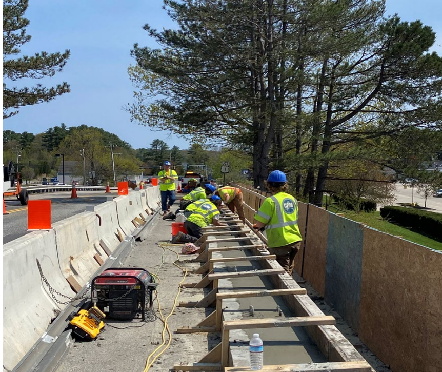
Concrete curb repairs at Wilson Road.
