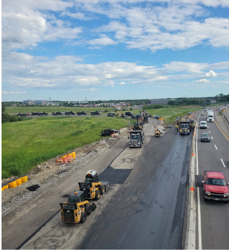
Paving mainline during the Exit 46 Shutdown
