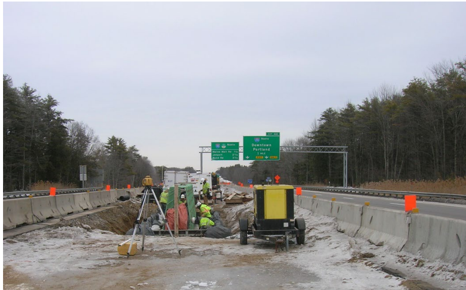
Constructing an overhead sign structure foundation in the median
