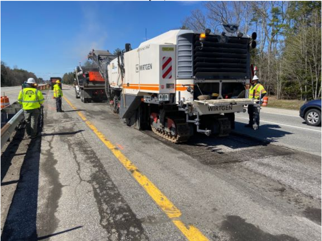
Pike Industries milling lane 1 at MM32.5 SB.
