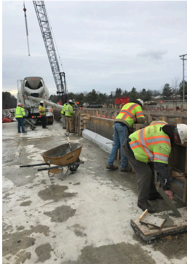
Placing concrete in parapet forms
