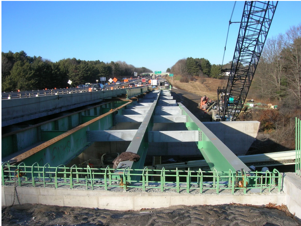
New structural steel at Stroudwater NB
