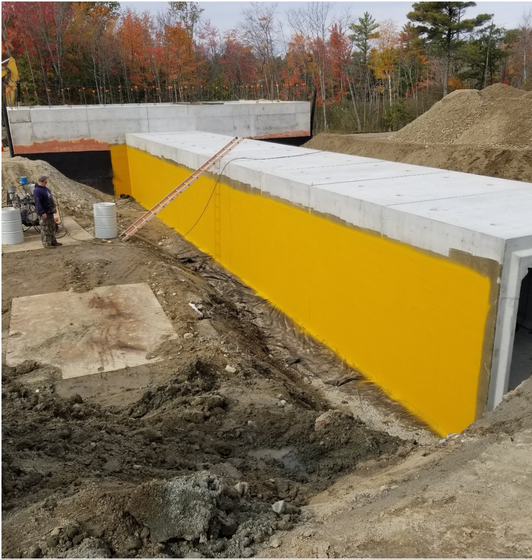
Admin building and phase 1 tunnel section, applying waterproof membrane
