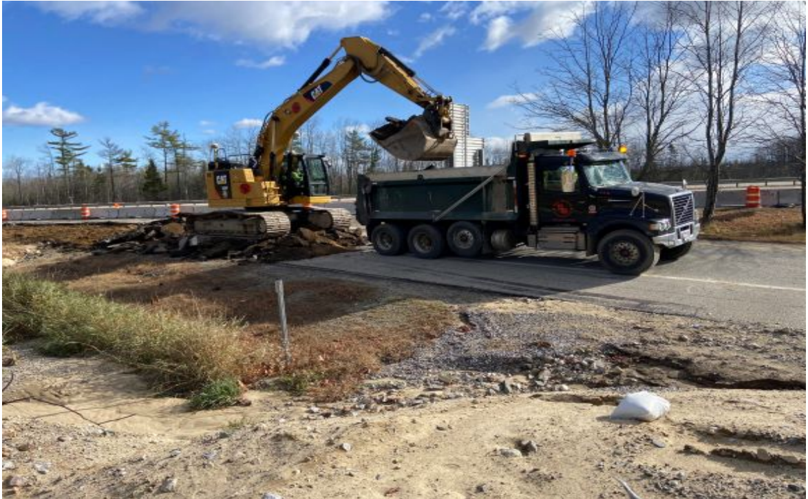
Shaw Brothers removing portions of the old South Bound off Ramp
