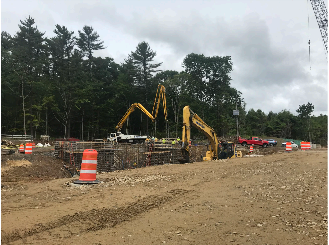
Foundation crew working on the toll administration building.
