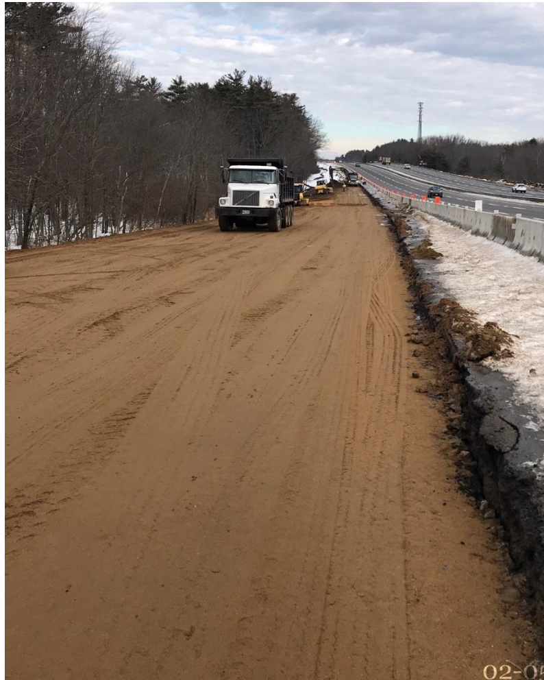
Box cutting shoulder and back filling with gravel
