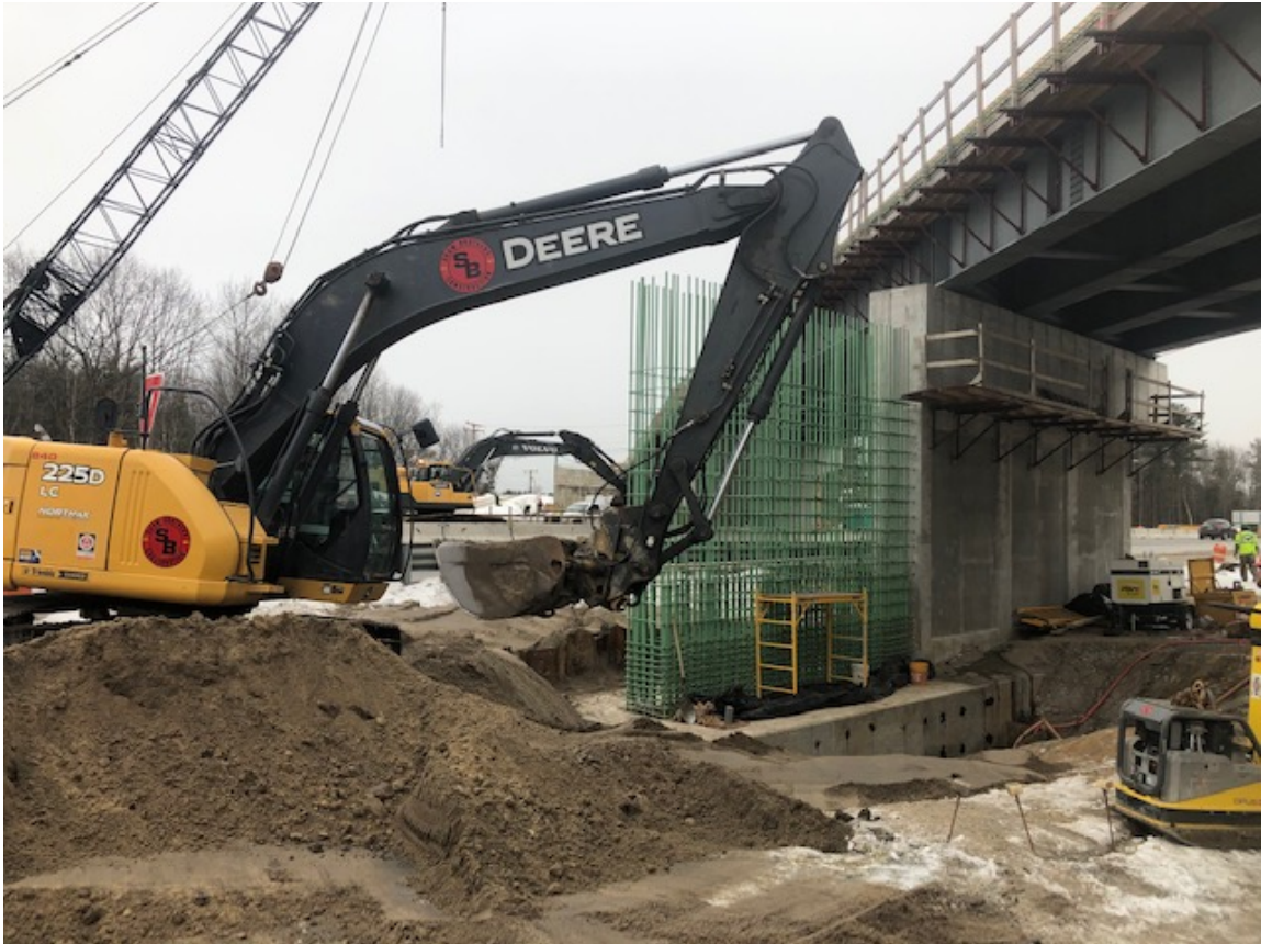
Pier 2 Stem wall reinforcing steel
