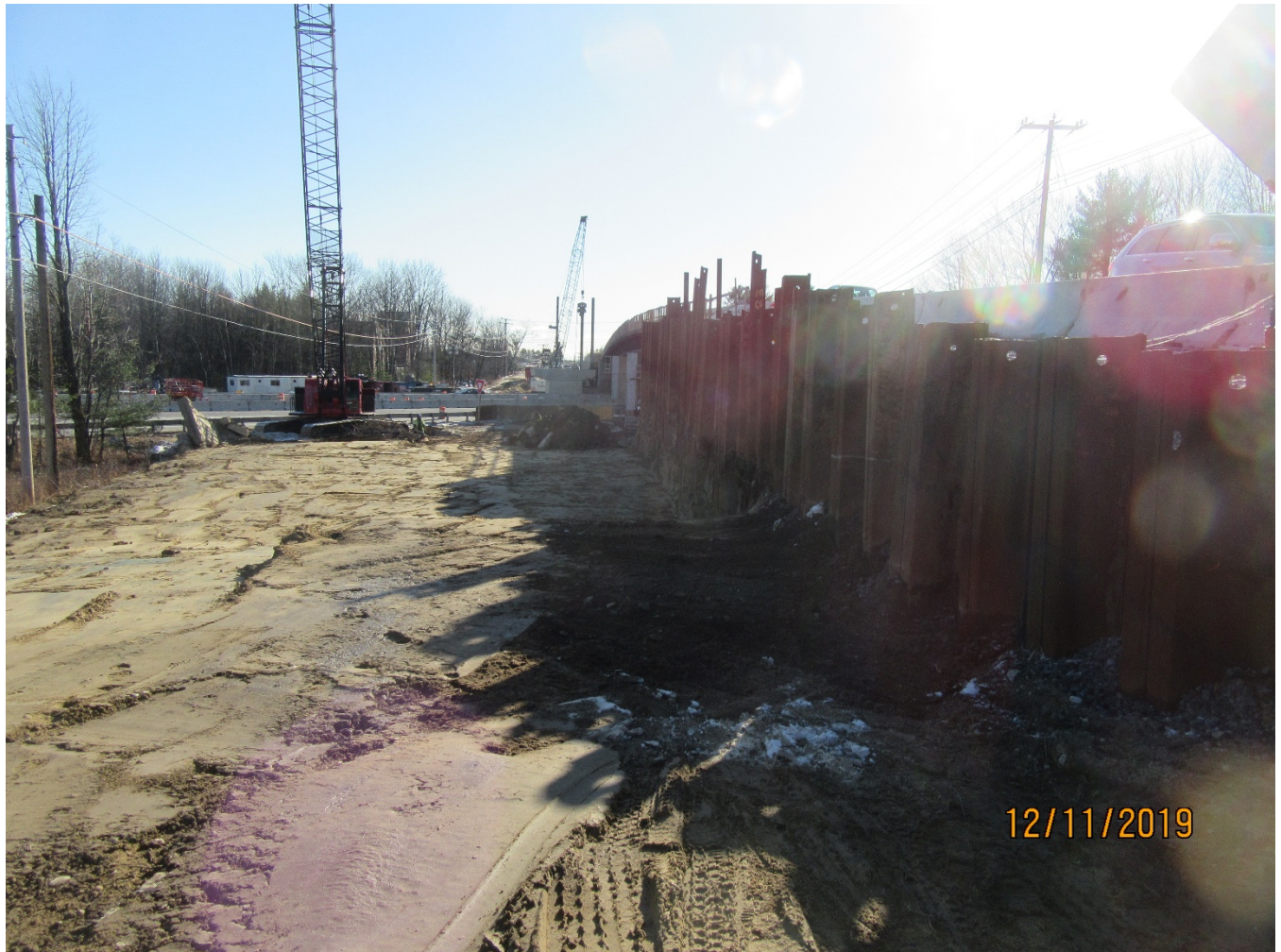
Existing bridge removed only pier 2 remains.
