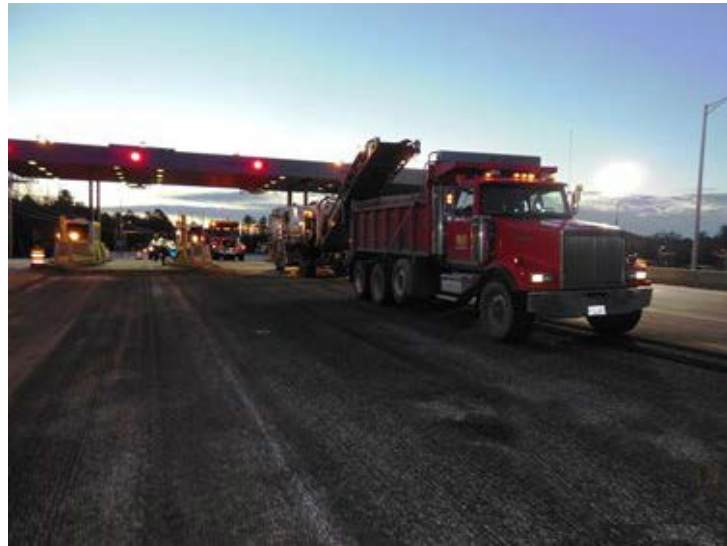
Paving crew milling pavement at Exit 42 early in the a.m.
