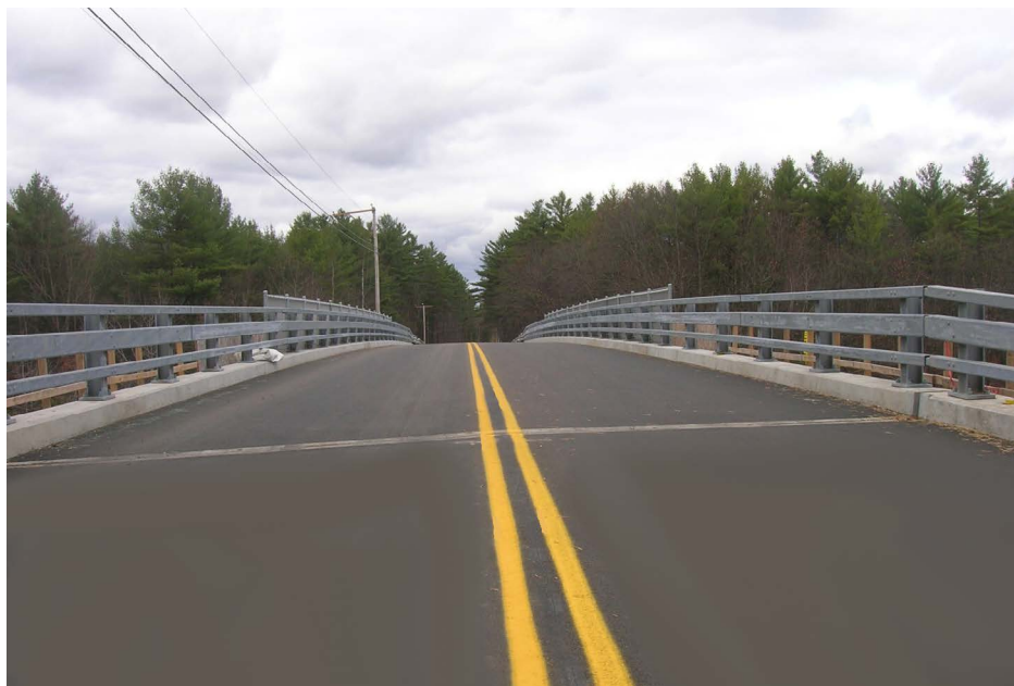
A view of Chandler Mill Road bridge after $1.3 million in rehabilitation.
